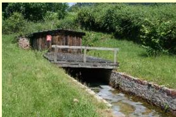
Mundloch des Mansfelder Schlüsselstollens
